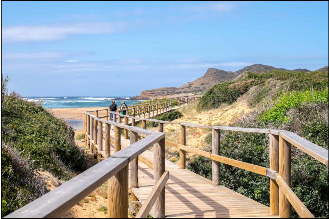
Figure 4-9: Elevated timber walkway.
