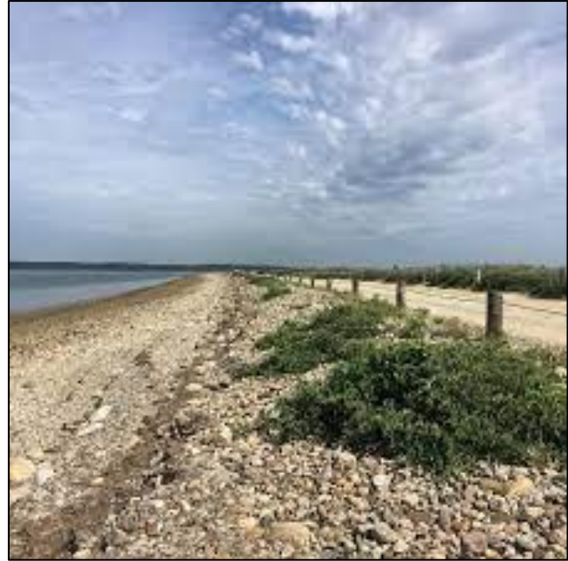
Figure 4-14: Vegetated cobble berm.
