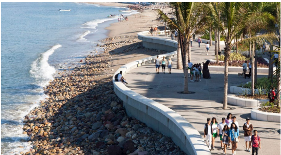
Seawall & Rock Revetment; Puerto Vallarta, Mexico
