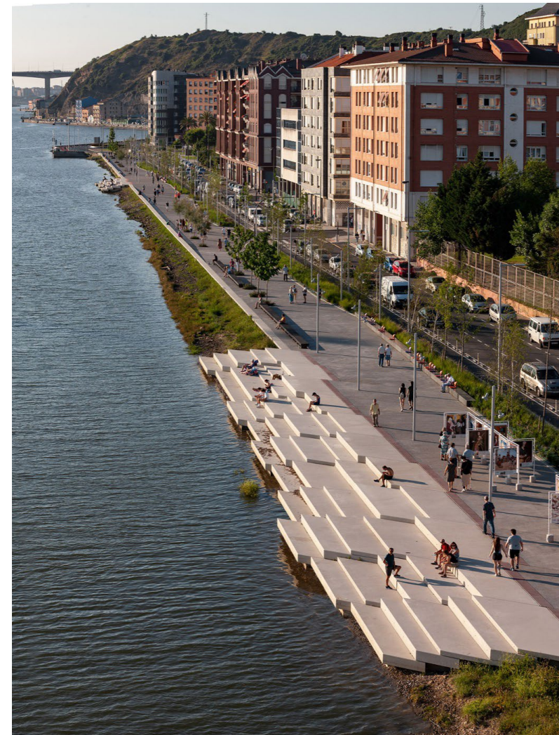
Fortified shoreline designed for public access
