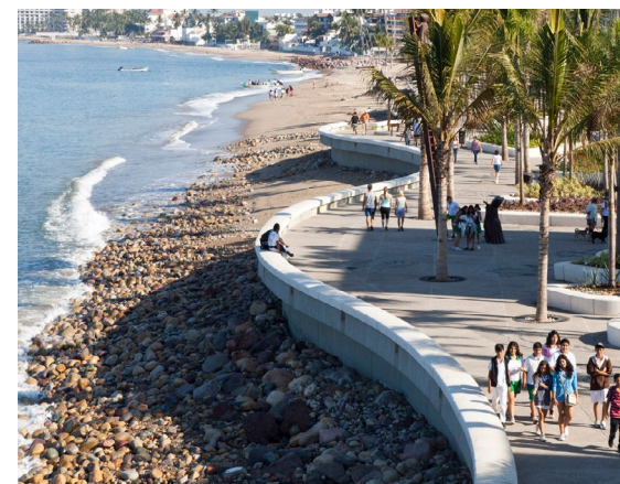
Concrete promenade and rock revetment Puerto Vallarta
