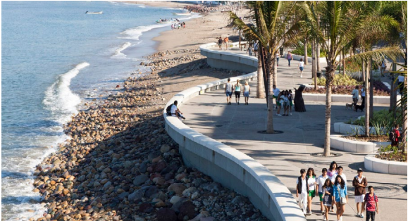
Seawall & Rock Revetment; Puerto Vallarta
